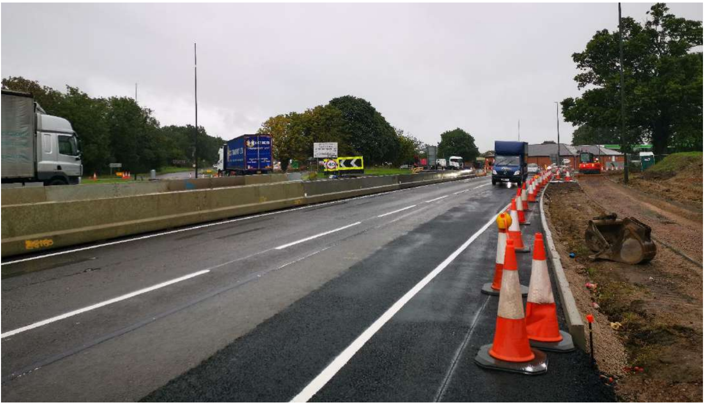
Barriers have been installed along the central reservation between the northbound/southbound arm of the A38 to/from Gloucester to protect our workforce.
