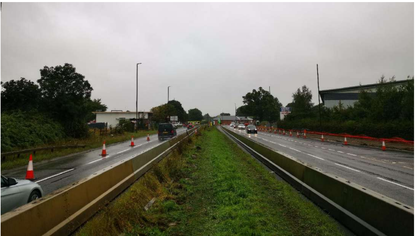
Barriers have been installed along the central reservation between the northbound/southbound arm of the A38 to/from Gloucester to protect our workforce.
