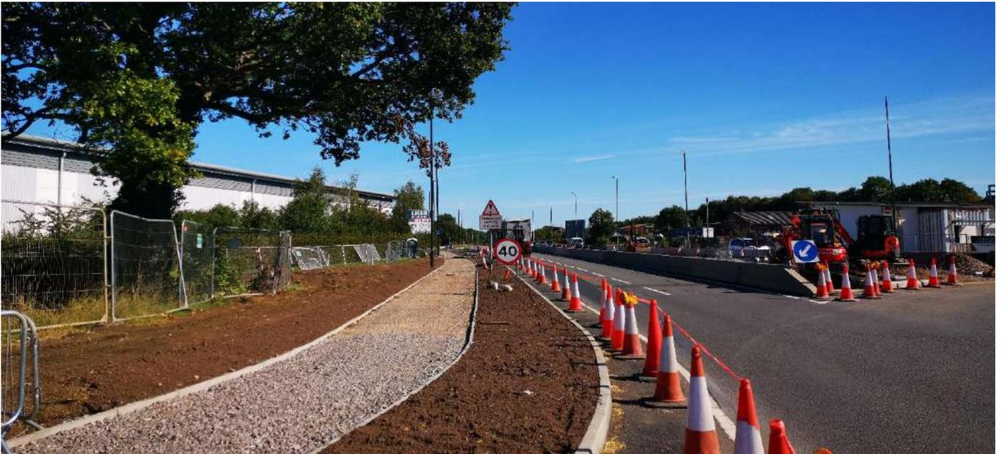
The central reservation between the A38 toward/from Gloucester is also well underway, with the new kerb line and sub-surface installed.
