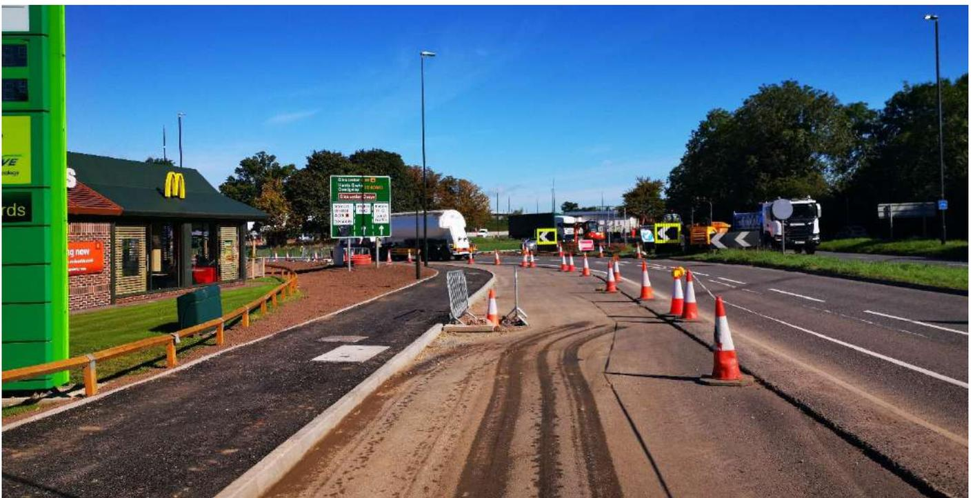
The footway on the A38 from the M5 (previously the B4008) has also been constructed, ready for the final surface course.
