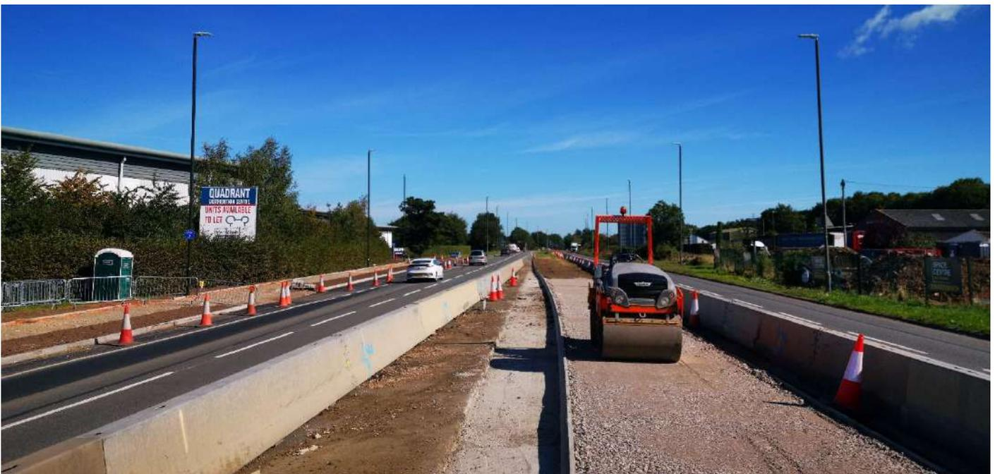
The central reservation on the A38 from/towards the M5 (previously the B4008) has been cleared, ready for the new kerbs and layout changes to be installed.
