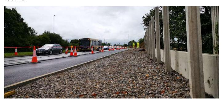
The island on the junction outside the services has been reconfigured and is prepared for the new surface.
