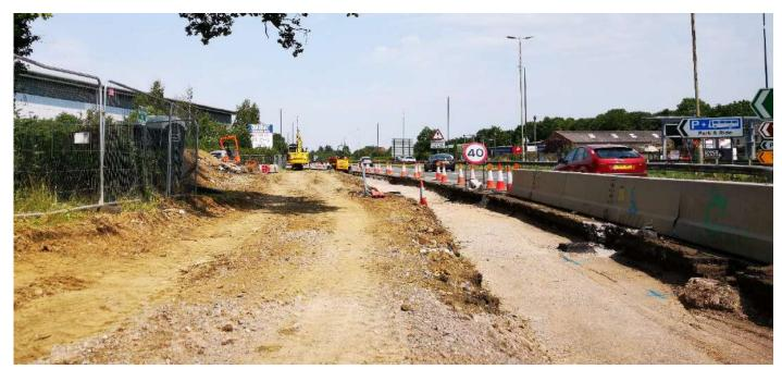
We have also completed the duct crossings we have been doing for the last two weeks on several junctions; the Bristol Road junction with the roundabout, the A38 to/from Whitminster/Stroud and both sections of the dual carriageway north of the roundabout heading to/from Gloucester.
