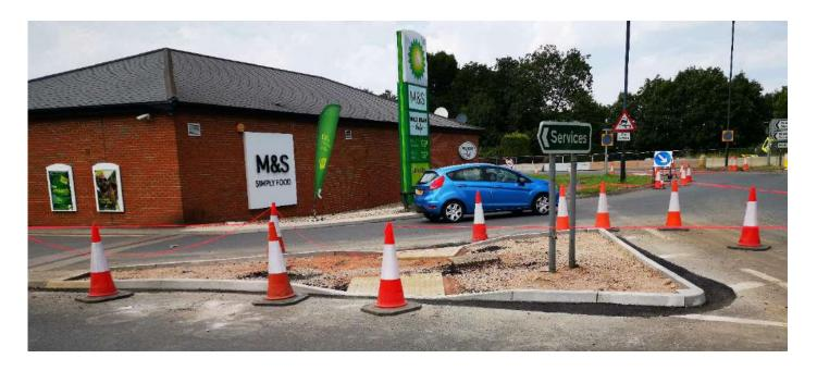
The drainage and kerbs will soon be complete where we are widening the carriageway as you head toward Whitminster/Stroud from Cross Keys Roundabout.
