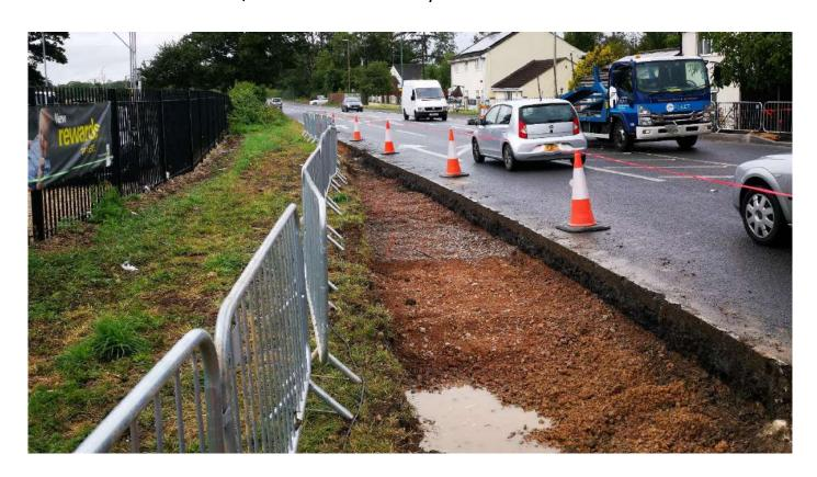
Works have continued in the verge between the A38 approach to Cross Keys Roundabout from Whitminster/Stroud and the A38 towards Gloucester from Cross Keys Roundabout, with the kerb alongside the new widened carriageway completed.
